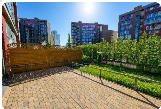
Large paved terrace
