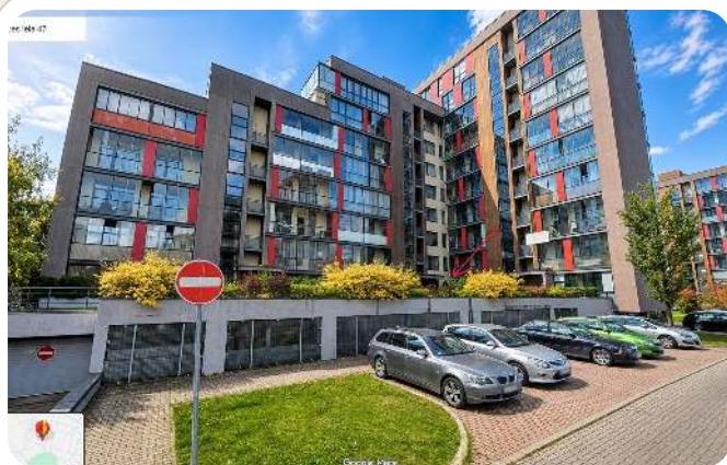
Entrance and parking
